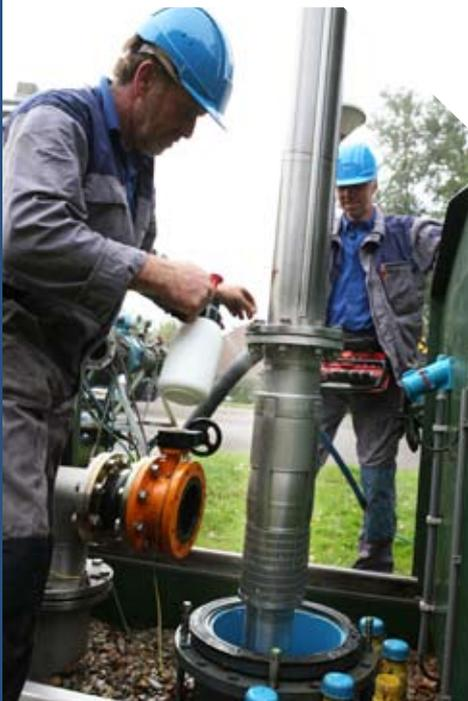
**Come together:** Vitens service technicians Drikus Geurtsen and Herman de Greeff install a new Grundfos SP submersible pump into a well at Loosdrecht. Below, De Greeff sprays the pump with chlorine to kill bacteria before lowering it. The seven Grundfos pumps better fit the flow demand of the well field, saving 21% energy. Right, Geurtsen empties the extraction pipe of water before removing the old pump.
